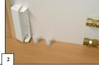
Any stretches under doorways should be done at the same time as the basic installation and positioned in the same way As for point. 1. NB: In large rooms there can be several connections, as the maximum circuit length for the heating panels should not exceed 15 metres. If there are empty pipes, cut them off level with the floor.
