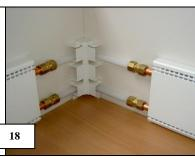
**Corners which are not 90°:** Place 2 blank panel brackets Type KA near the corner. Cit the blank panels with a bevel.
